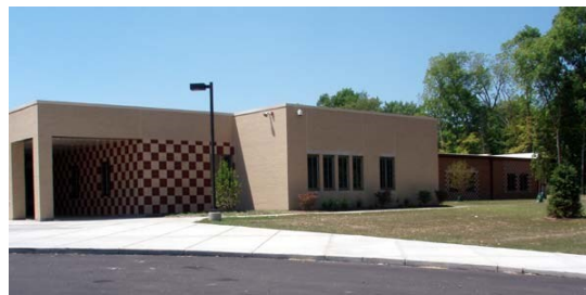
Westbrooke Village Elementary School
